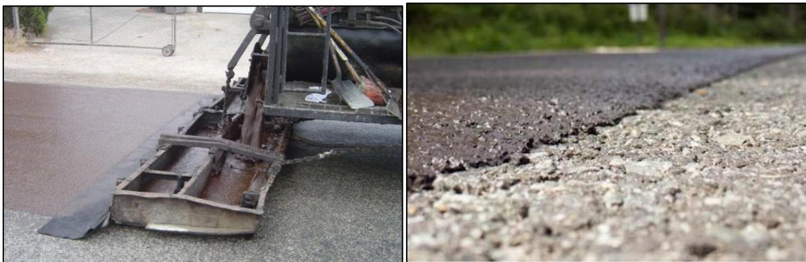
Figure 23. Spreading of Micro-surface Slurry
