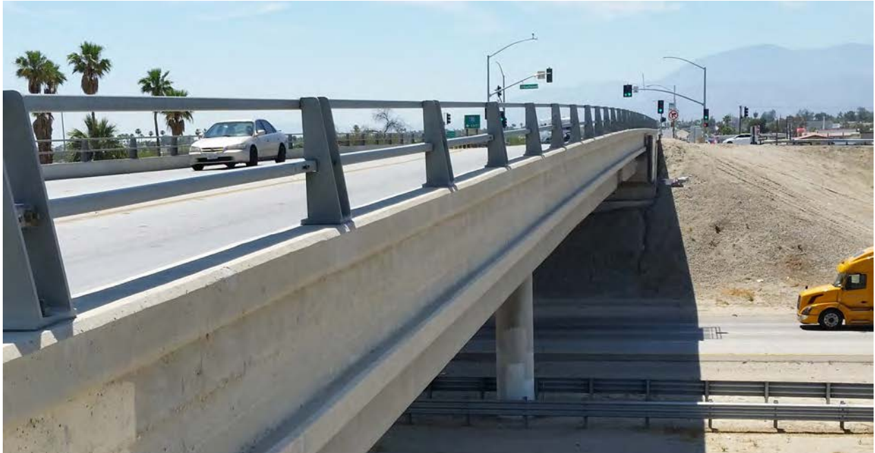
Photograph No. 1: View of bridge along Monroe Street over I-10 freeway facing north.
