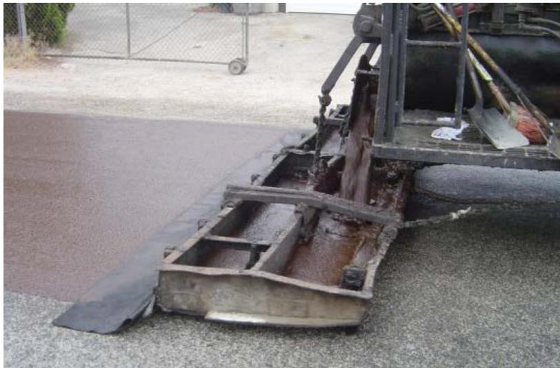
**Figure 17. Spreading of slurry**
