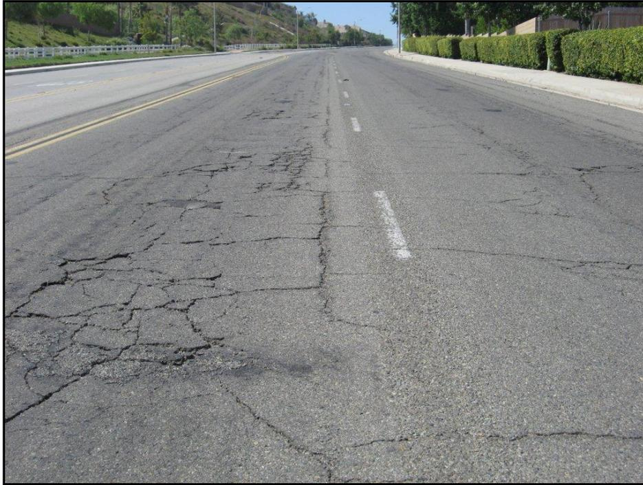
**Figure 2E. PCI=30 (Poor Condition)**
