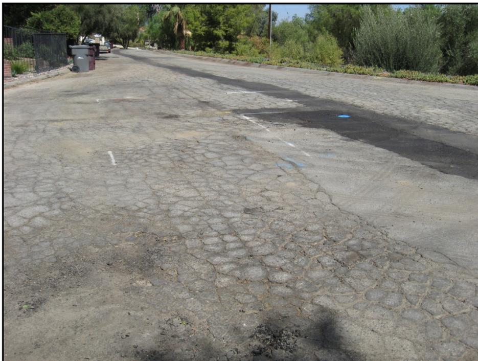
**Figure 2F. PCI<10 (Very Poor Condition)**
