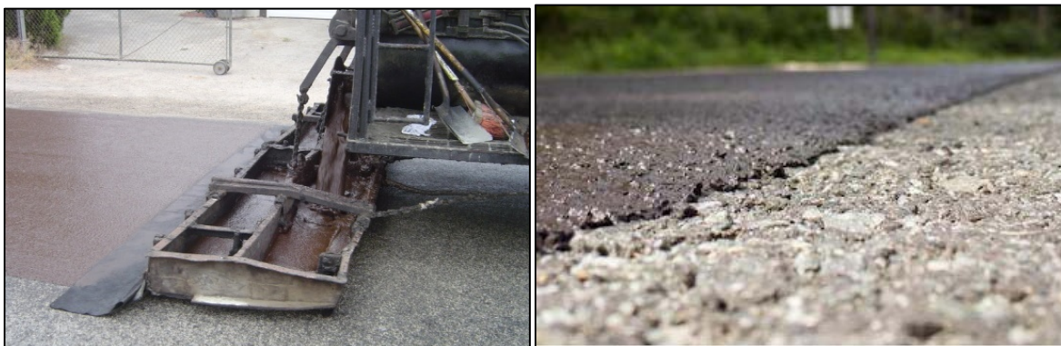
Figure 23. Spreading of Micro-surface Slurry
