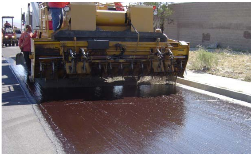
Figure 16. Spreading of chip over emulsion
