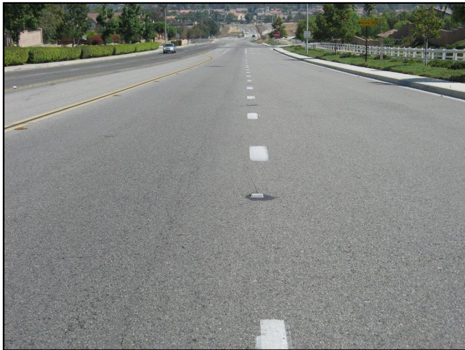
Figure 2B. PCI=85 (Very Good Condition)
