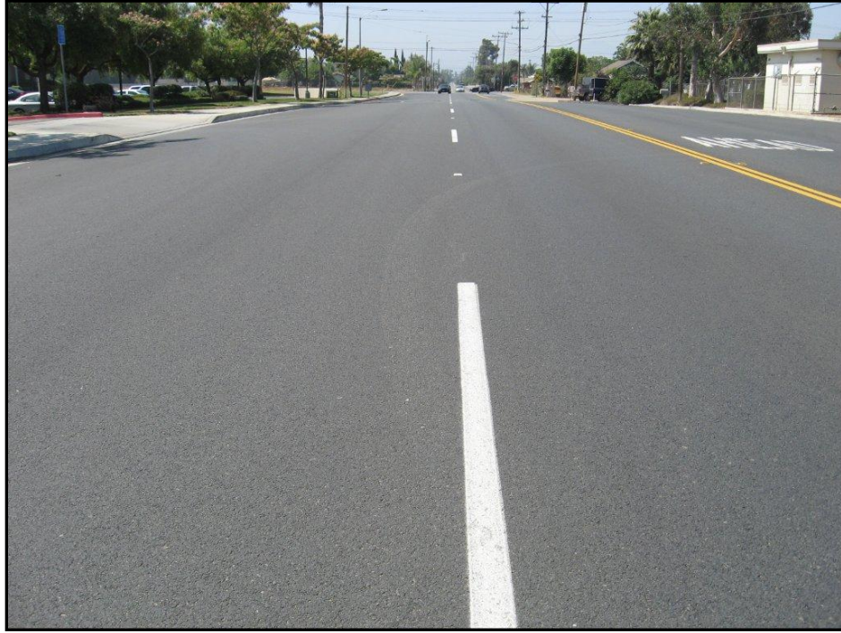
Figure 2A. PCI=98 (Excellent Condition)
