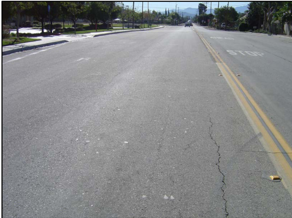
Figure 2C. PCI=78 (Good Condition)
