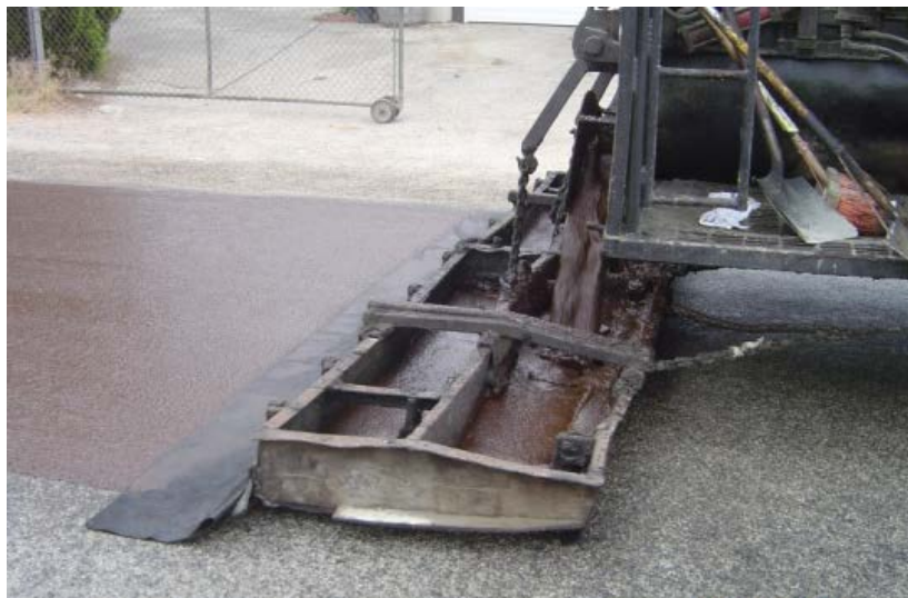
Figure 17. Spreading of slurry
