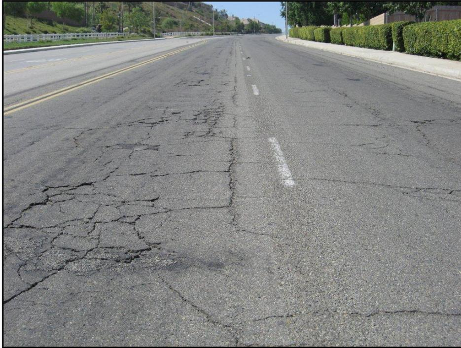
**Figure 8E. PCI=30 (Poor Condition)**
