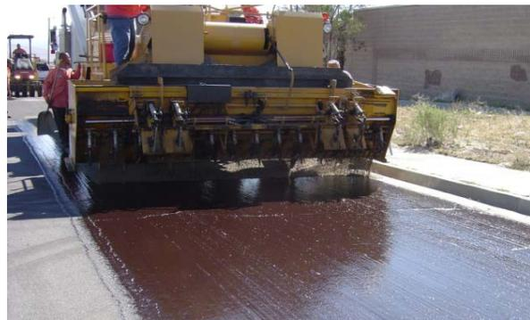
**Figure 16. Spreading of chip over emulsion.**
