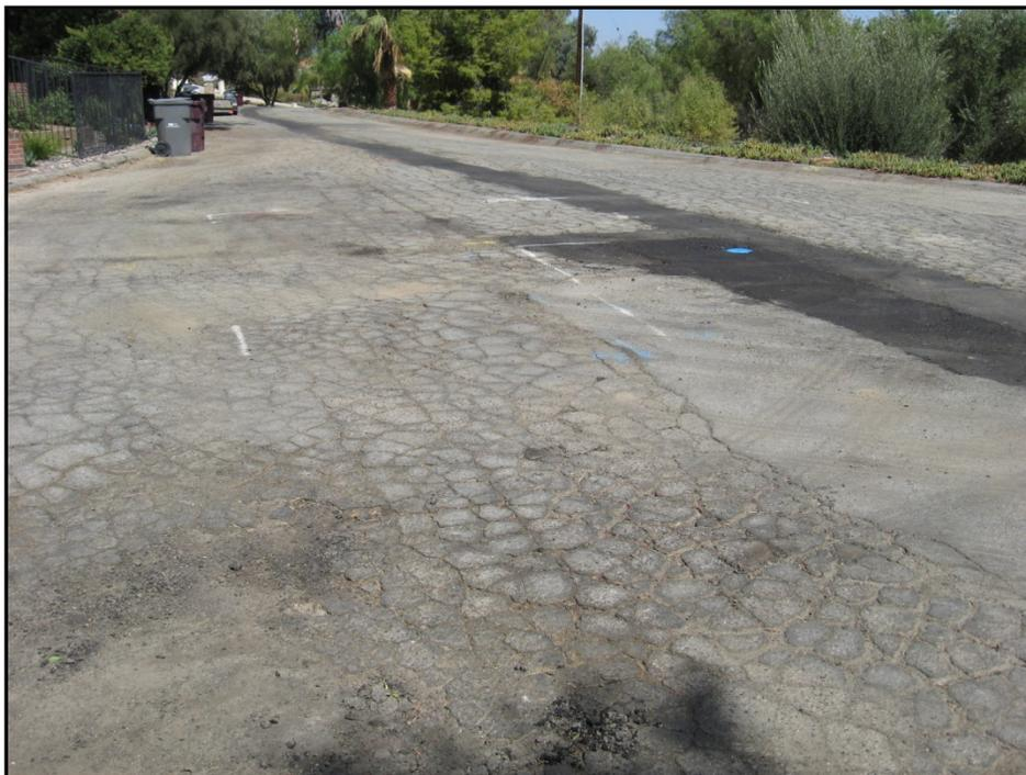
**Figure 8F. PCI<10 (Very Poor Condition)**
