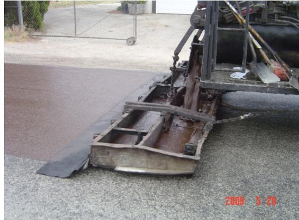
**Figure 17. Spreading of slurry.**
