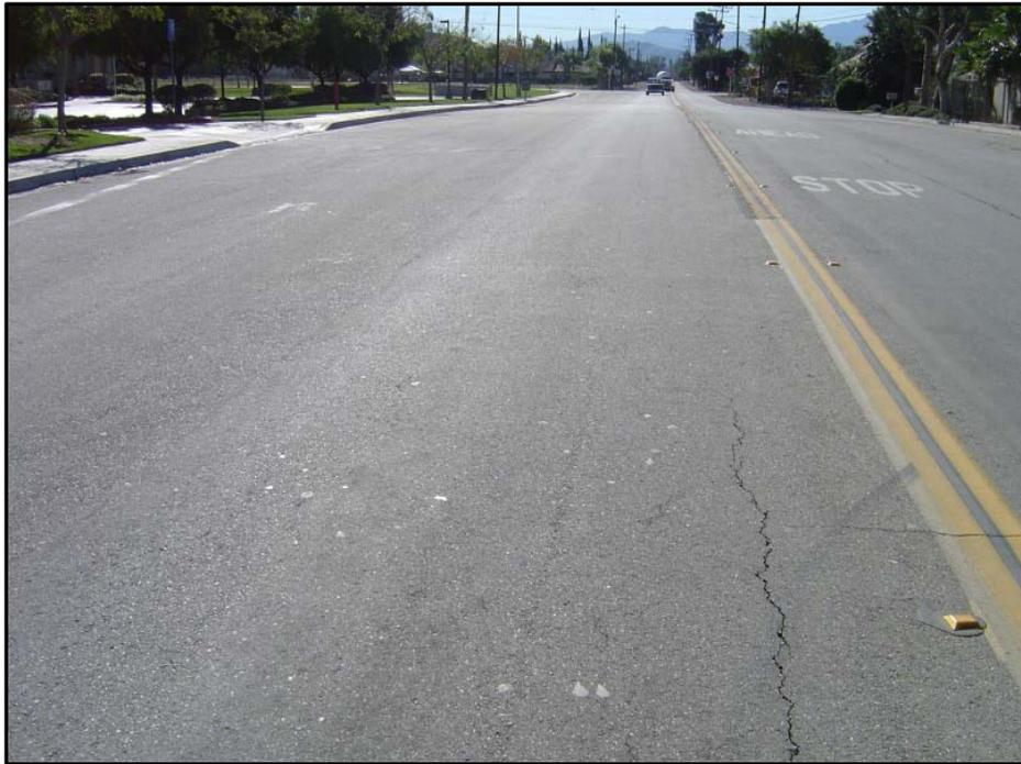
**Figure 8C. PCI=78 (Good Condition)**
