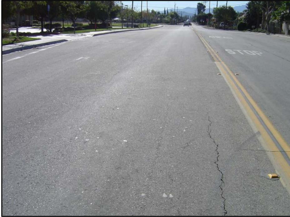
**Figure 8C. PCI=78 (Good Condition)**
