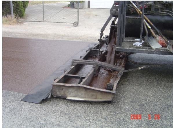
Figure 20. Spreading of slurry.
