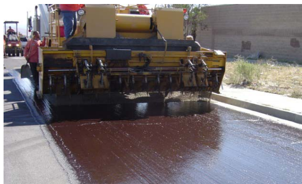
Figure 19. Spreading of chip over emulsion.
