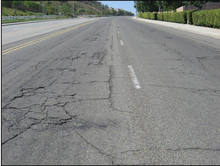
**Figure 2E. PCI=30 (Poor Condition)**
