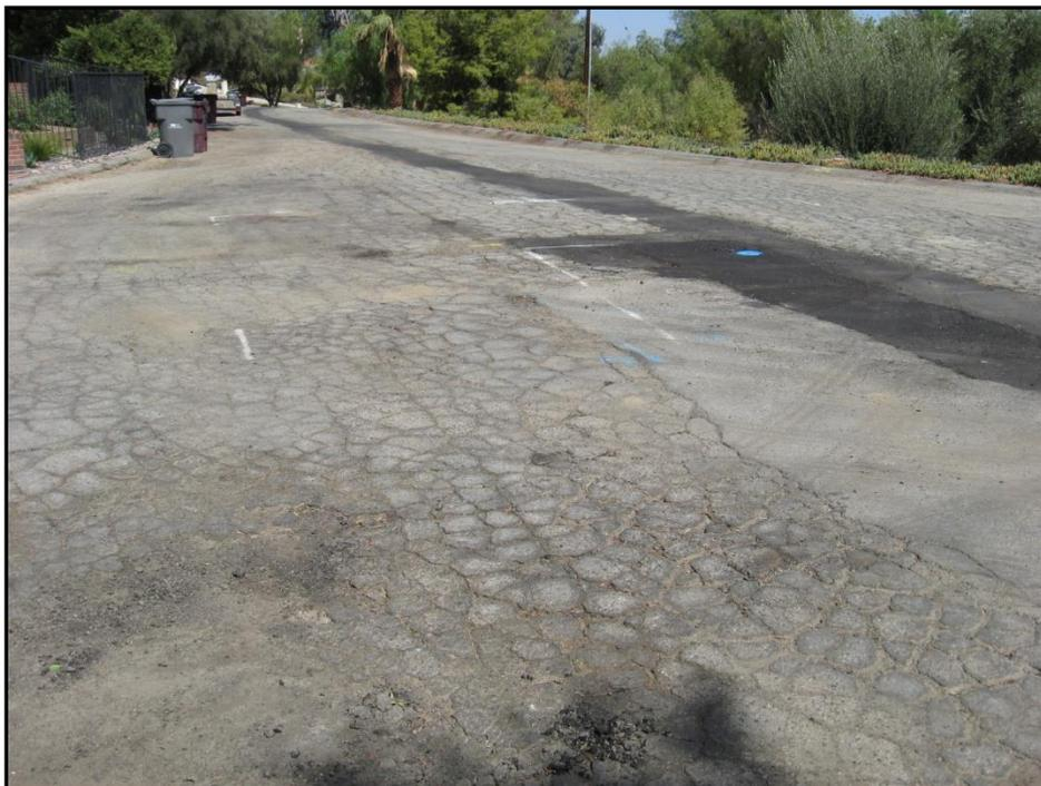
**Figure 2F. PCI<10 (Very Poor Condition)**
