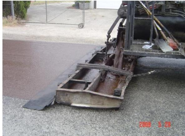
**Figure 19. Spreading of slurry.**
