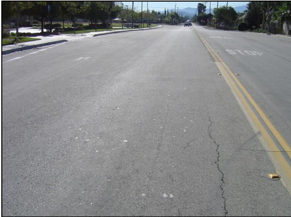
**Figure 2C. PCI=78 (Good Condition)**
