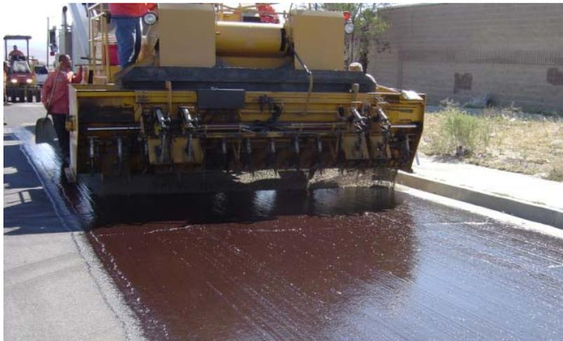
**Figure 16. Spreading of chip over emulsion**
