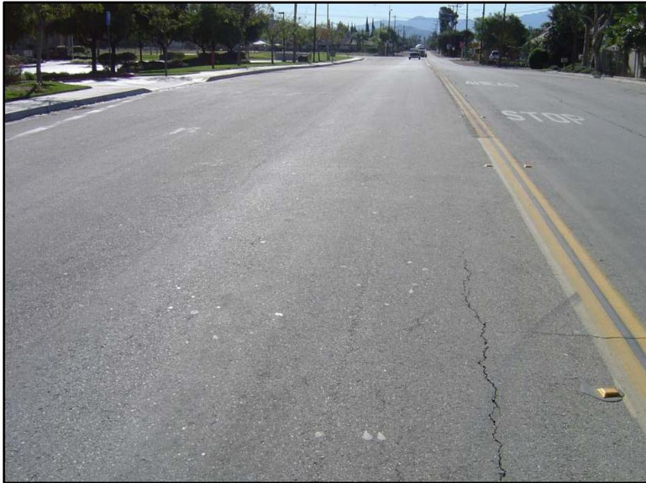
**Figure 2C. PCI=78 (Good Condition)**
