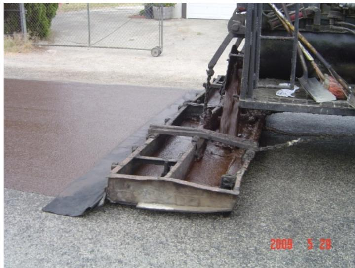
**Figure 17. Spreading of slurry**
