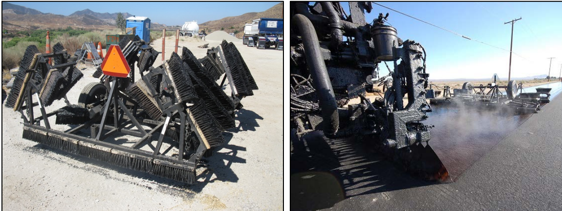
Figure 22. Scrub Seal (brooms on left, in use on right)
