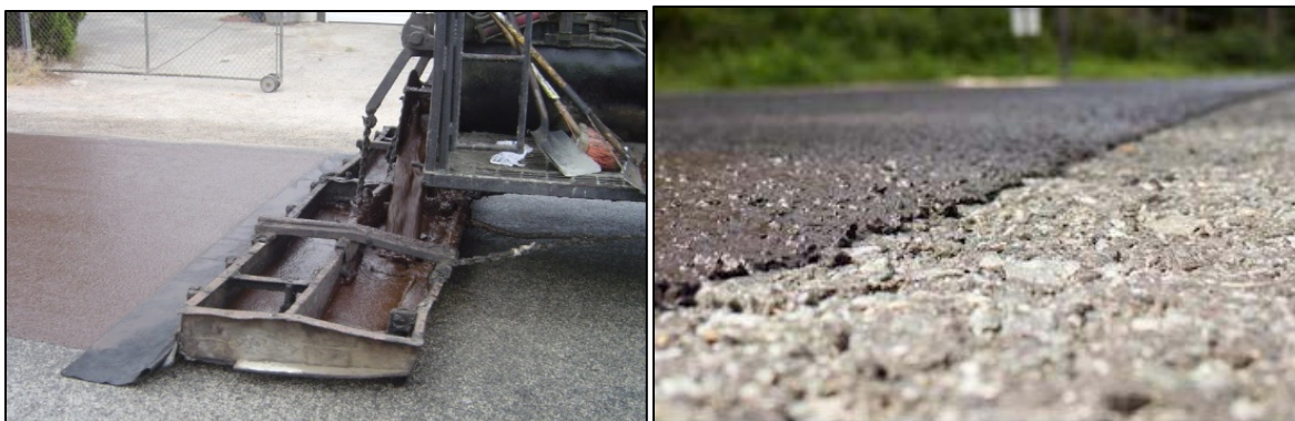
Figure 23. Spreading of Microsurface Slurry
