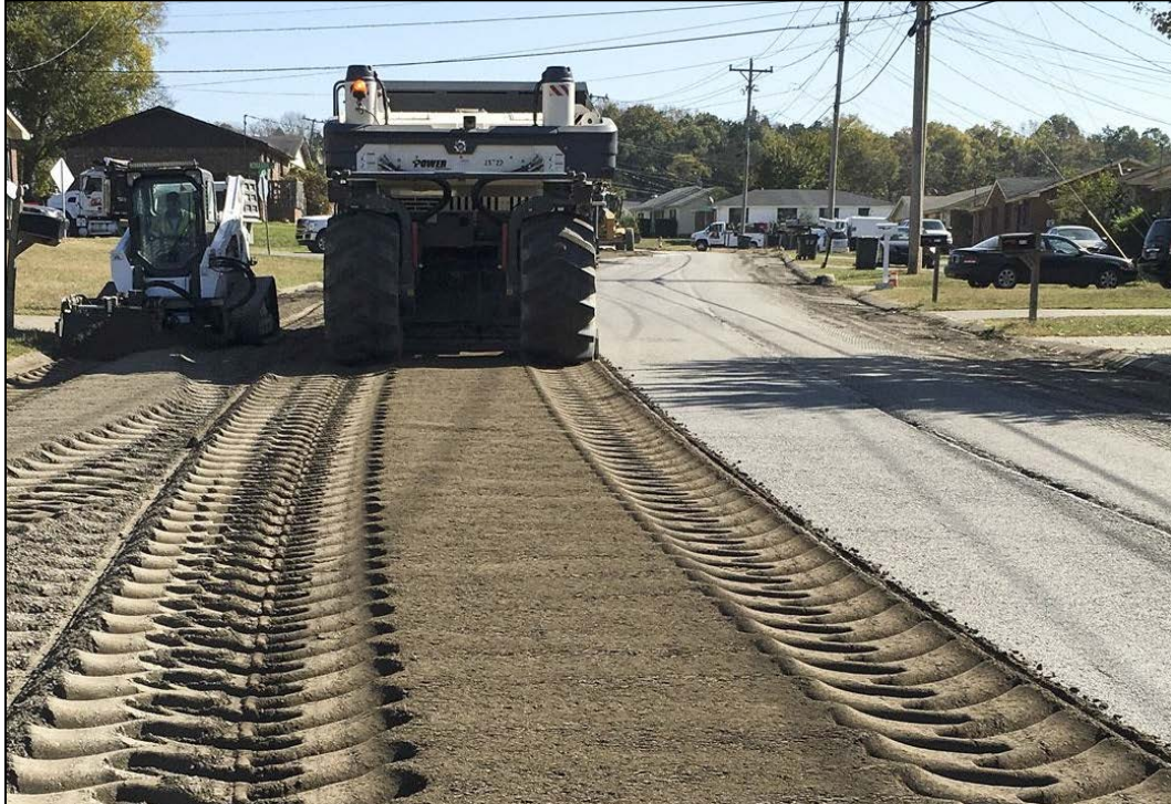
Figure 26. Full Depth Reclamation (FDR)
