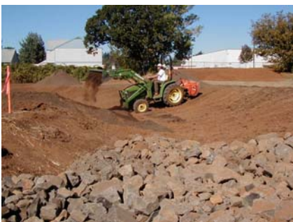
Soil is prepped for better plant growing conditions
